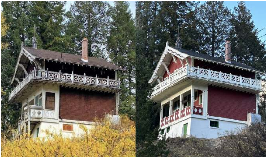
1 The Edward Feuz Chalet pre- and post-renovations of the exterior undertaken by the new owner, Montayne (photo: Remax/I.Spaar)
